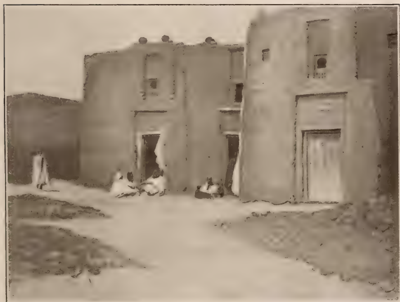
Laing's house, Timboctu.
